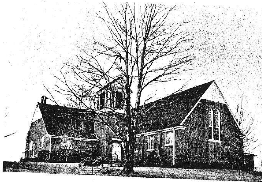
Exterior of Mooresburg Presbyterian Church
